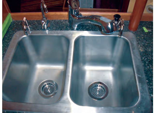
The double sink
